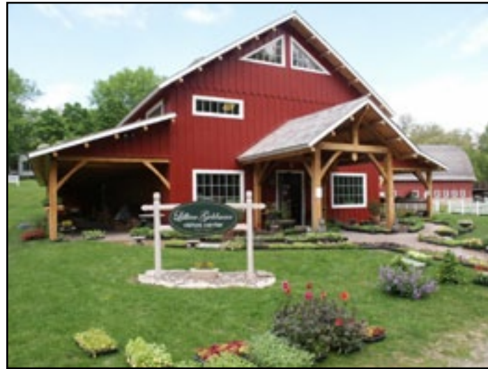
Above and left: The Heritage Farm barn was restored by Amish carpenters and serves primarily as a conference center in the summer and a storage facility in the winter. The Lillian Goldman Visitors Center houses educational displays, artwork, and the Seed Savers store, and also provides sheltered space on its dual side porches for festive outdoor events. (SSE photos)
