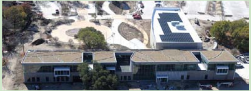
North view of the BRIT Campus looking south.
